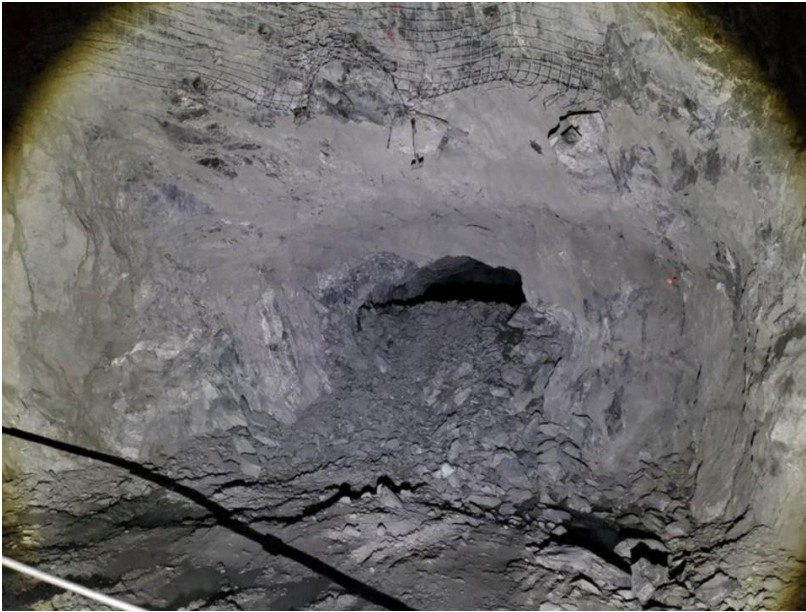
North cavern breakthrough January 2022
