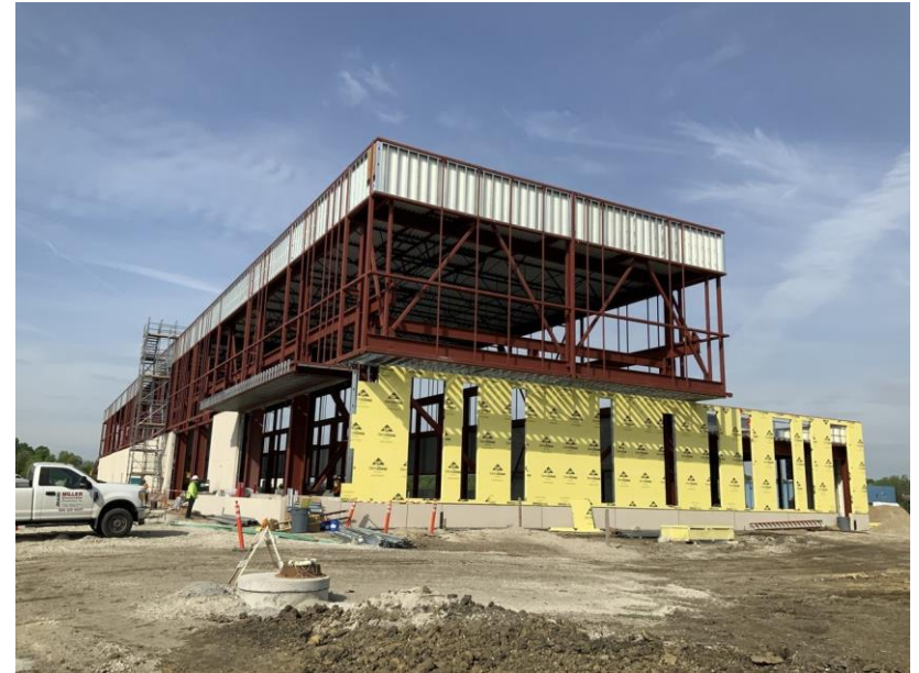
PIP-II construction May 2022
